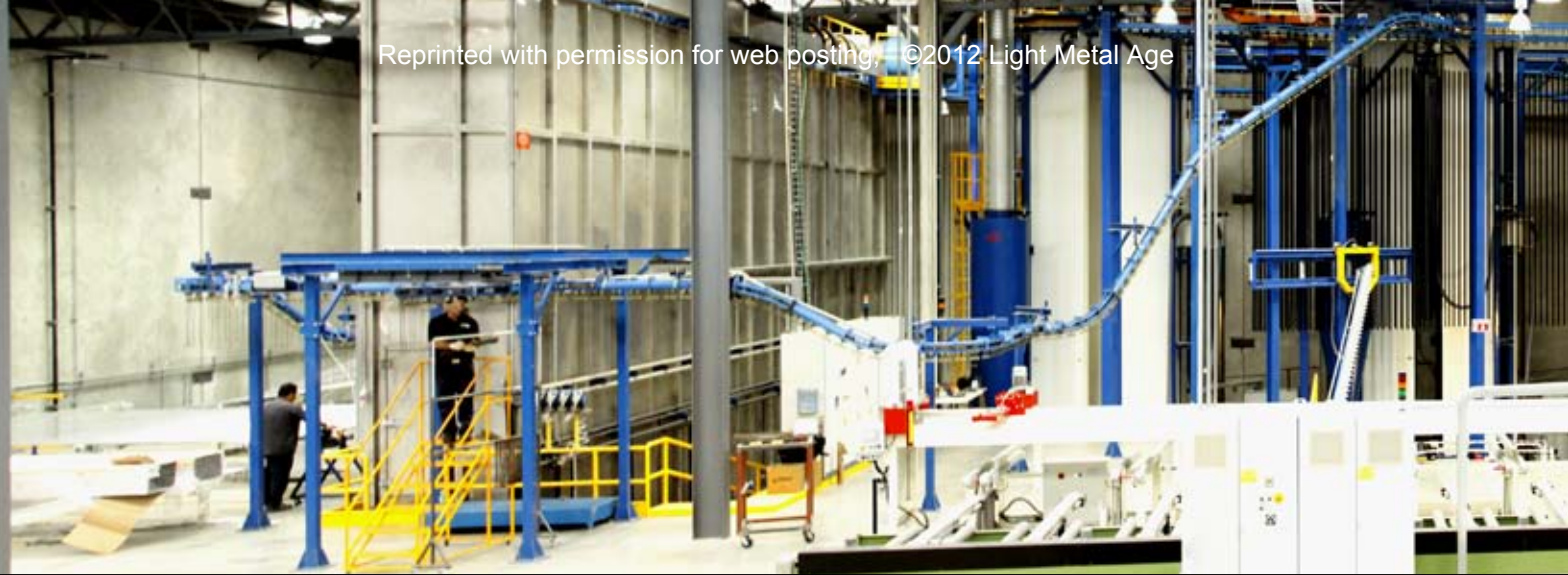
Figure 1. Panoramic view of powder coating: (L-R) loading, pretreatment, powder application, curing, and sawing.
